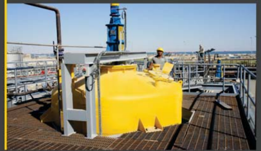
40 KL FRP Reaction vessel with agitator assembly mounted separately
