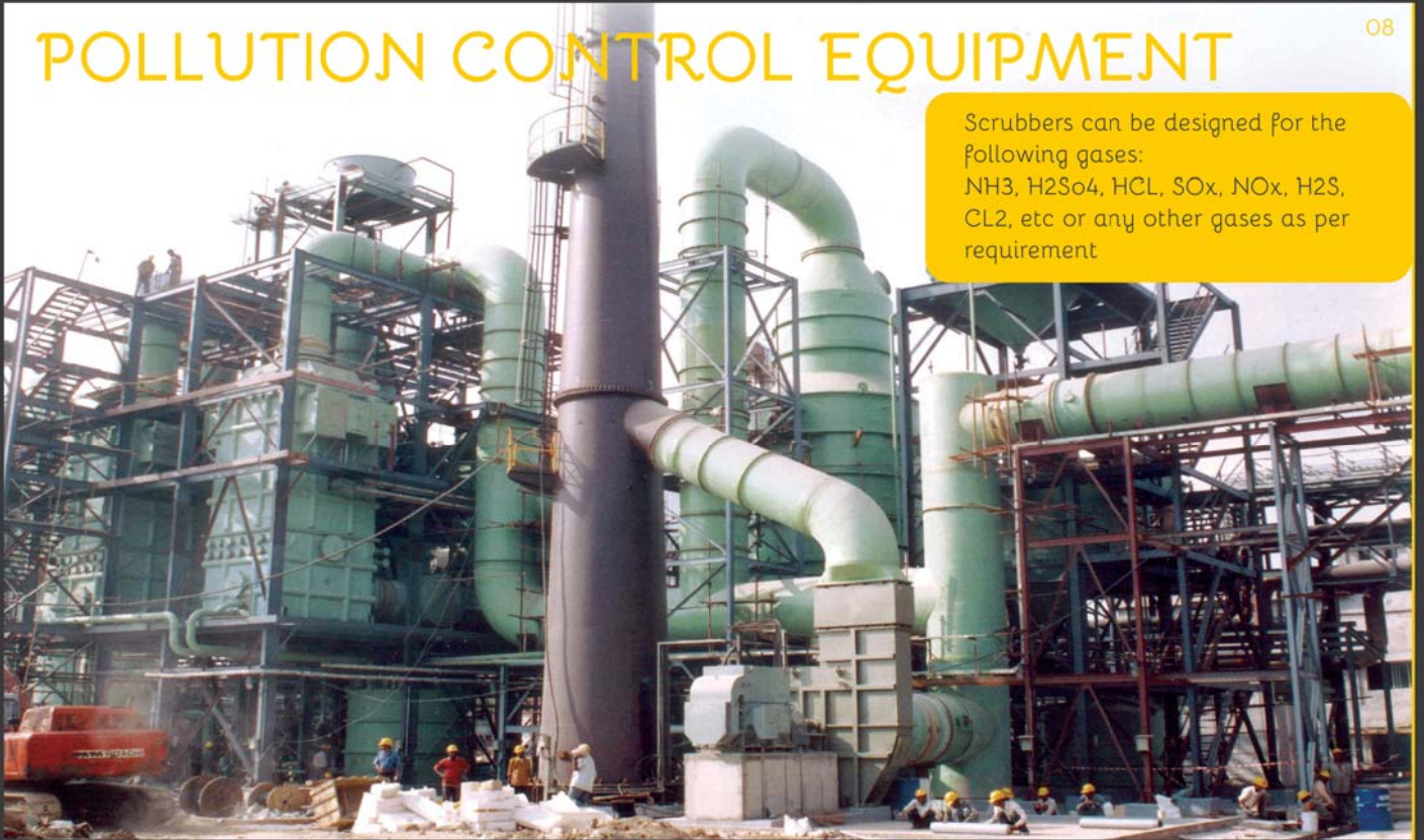
Mercury removal tower 5.3 m Dia x 18.4 m Height
